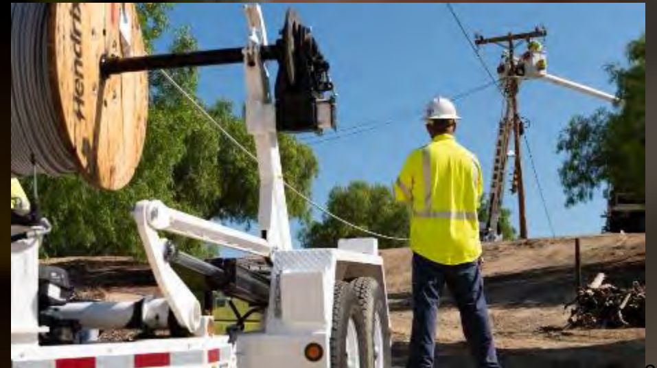
Above photos: SCE crew installing insulated wire
