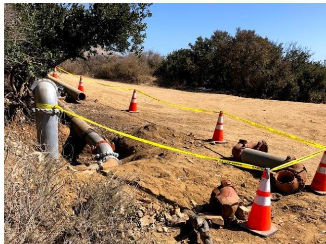
On August 10, Cal Water continued to repair damage caused to the nearby fire hydrant on Burchell Lane and Crenshaw Boulevard on July 17. Repair work includes use of a backhoe to fill in and level the grade dip on Burma Road Trail, and clearing sediment buildup in an 8-inch pipe along Gary's Gulch Trail.
