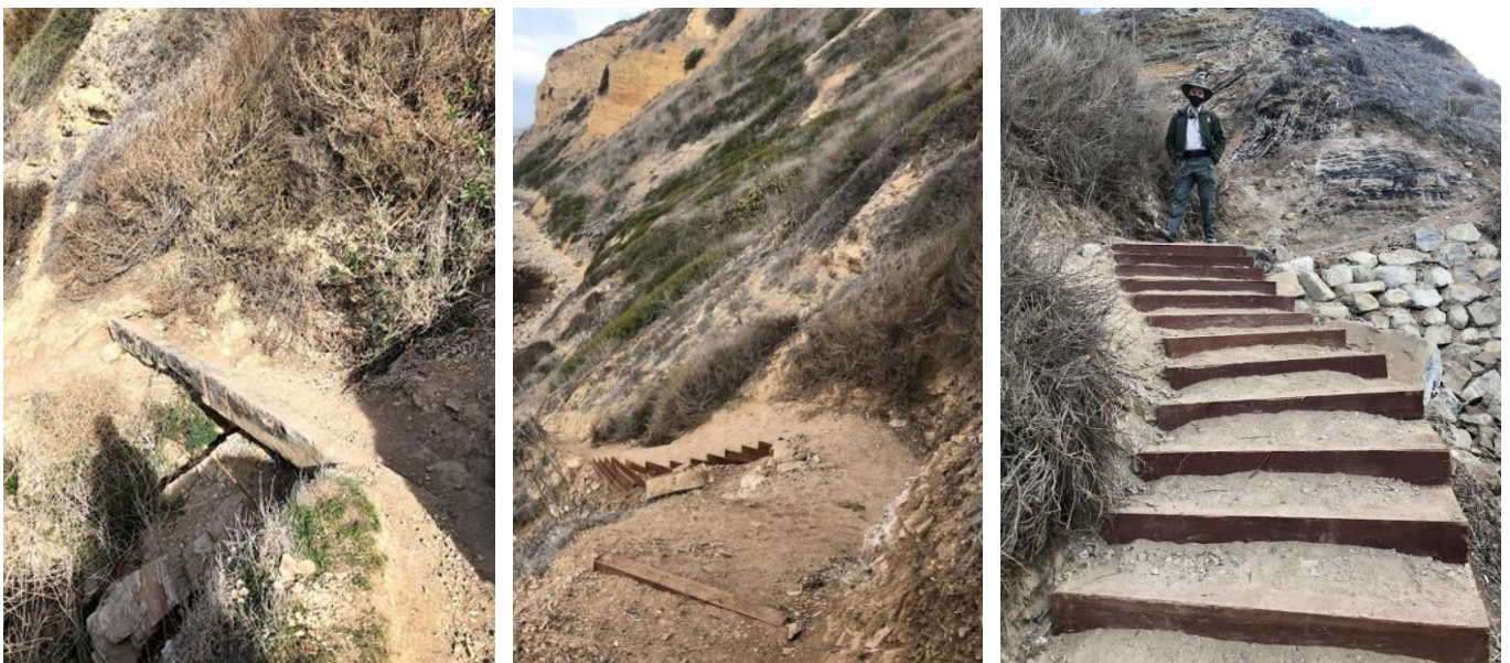
Two sets of timber box steps were installed on the upper and middle sections of Southshore Coastal Trail, among other improvements, to assist with water control measures. The image on the left was taken in February 2021. The center and right images were taken in November 2021 in the same location from different angles.
