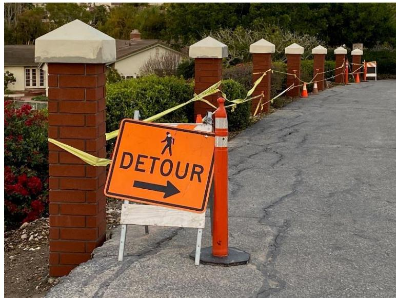
Modifications to the bollards at the Burma fence and gate are expected to take 2-3 weeks. The final configuration will consist of one fixed bollard at each end and three removal bollards in the middle. The project is anticipated to be completed by the end of January 2023.
