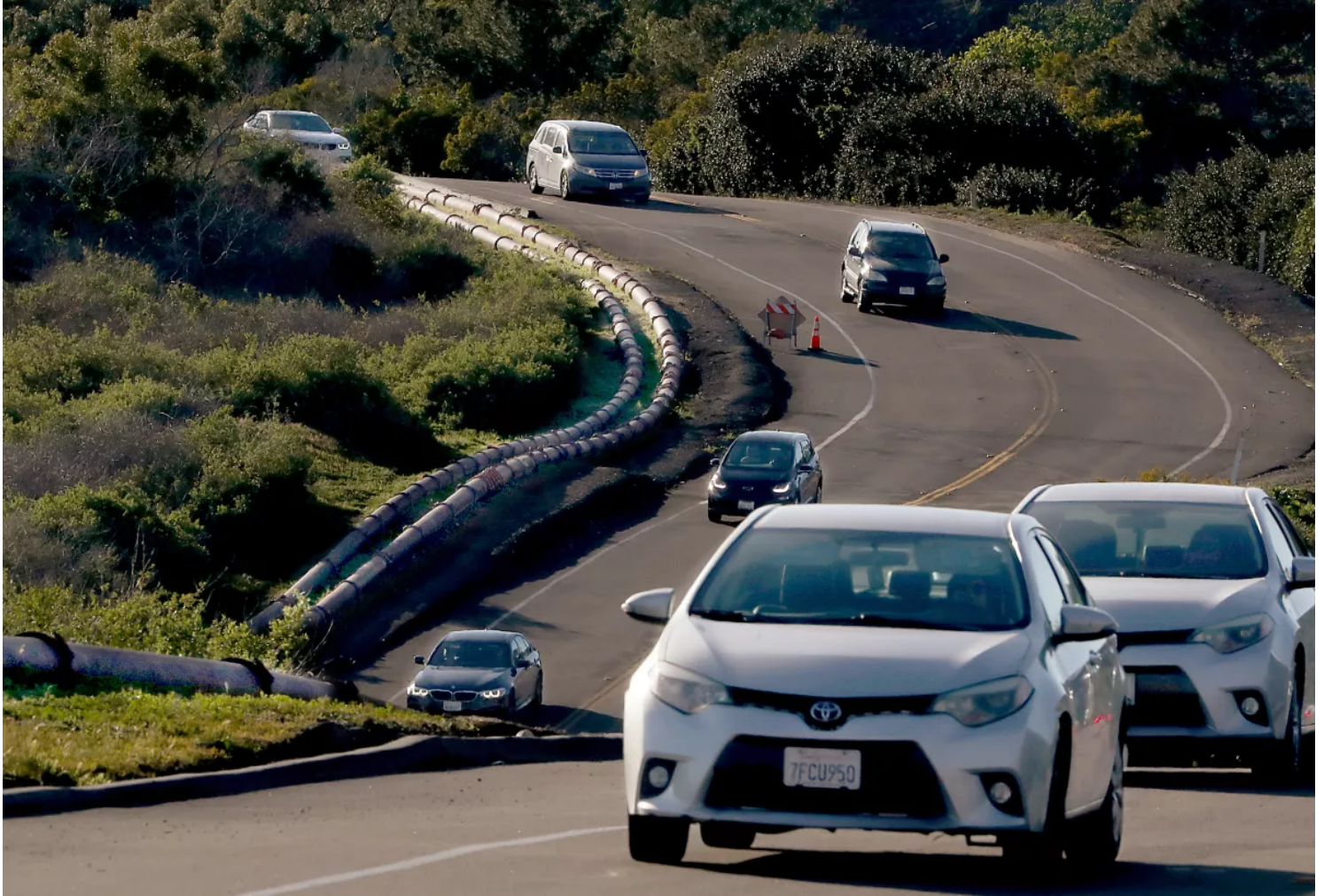
Sewage pipes run above ground along Palos Verdes Drive South at Portuguese Bend, where a stretch of roadway is uneven and erratic because of land movement on the coastline. (Luis Sinco / Los Angeles Times)
