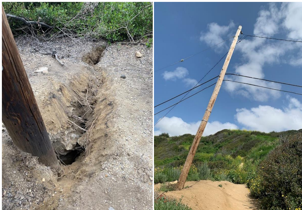
SCE infrastructure impacted by fissures/land movement
