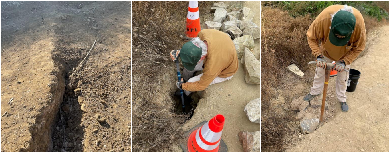
Local trail expert, Kurt Loheit, shows OSM some fissure filling techniques on fire roads within the Preserve.
