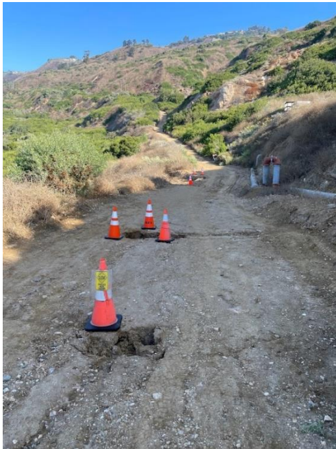
Before picture (left) was taken on August 25 with cones placed around the opened fissures compared to the picture after repairs (right) taken on August 28.
