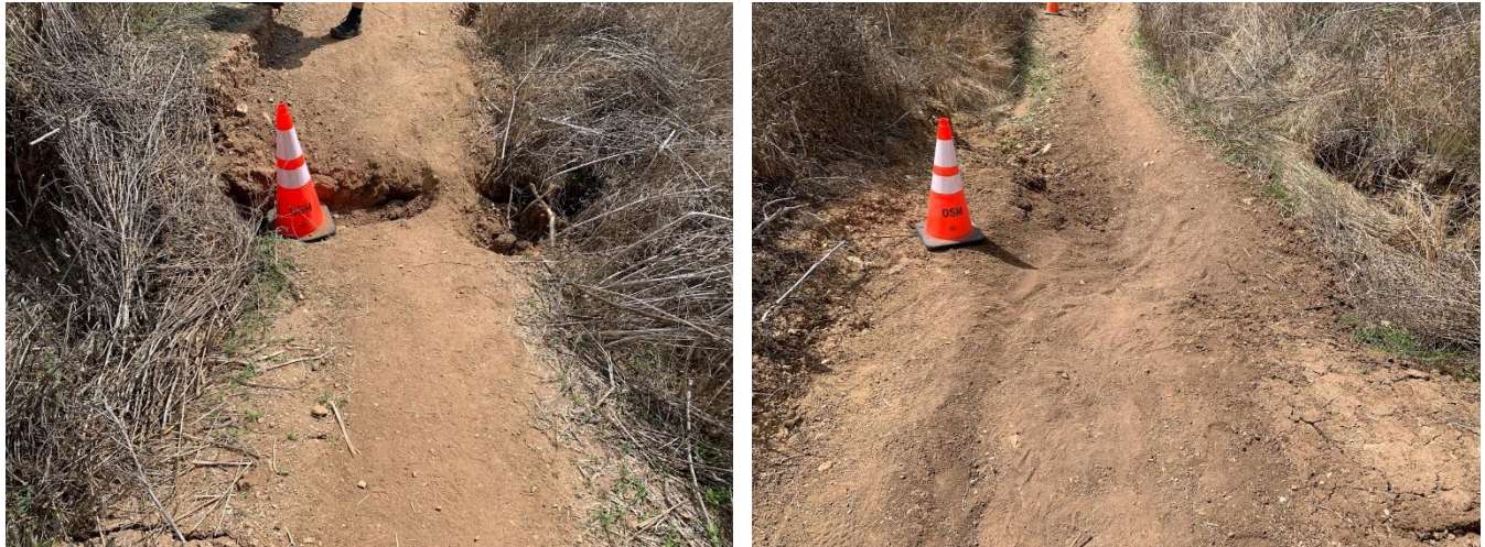
Before and after picture of fissure located on Klondike Canyon Trail.
