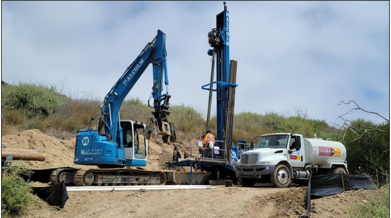
Drilling operations at the second borehole location
