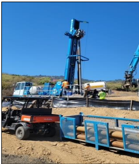
Drilling Operations at E-1-6 Seaward of Palos Verdes Drive South
