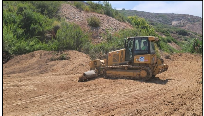
Borehole access route grading landward of Palos Verdes Drive South
