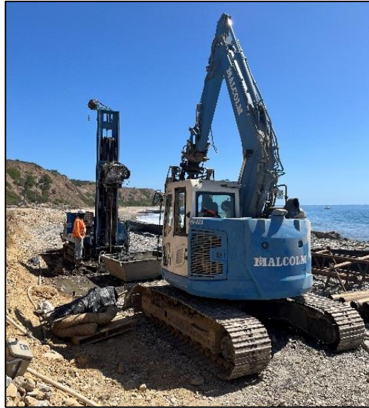
Drilling of the third dewatering well seaward of Palos Verdes Drive South
