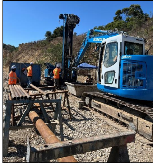
B. Installation of the Fifth Dewatering Well at the Beach
