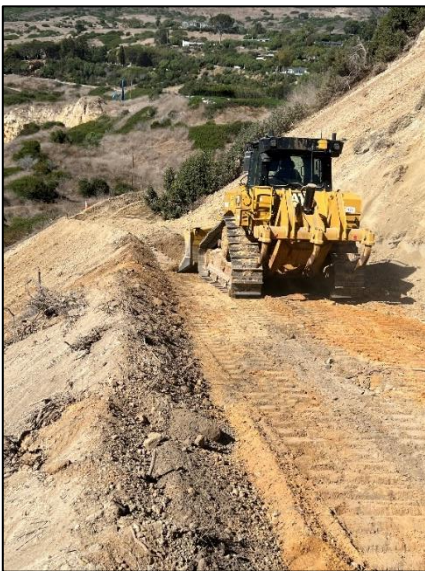
Development of Access Path to DDW-11 at Abalone Cove Beach (Left) and Fissure-Filling Work West of Altamira Canyon (Right)
