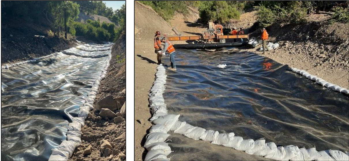
Installation of Temporary Liner at the Base of Altamira Canyon
