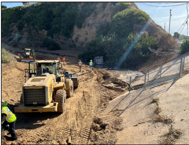
Grading of the Detention Pond at the Base of Klondike Canyon (Left) and Completed Lining of Klondike Canyon (Right)
