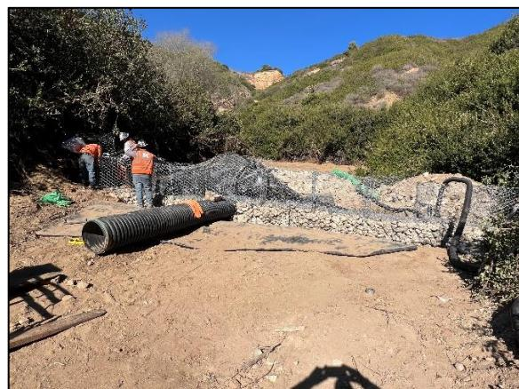
*Installation of New Gabion and Drainage Pipe in the Upper Section of Klondike Canyon*
