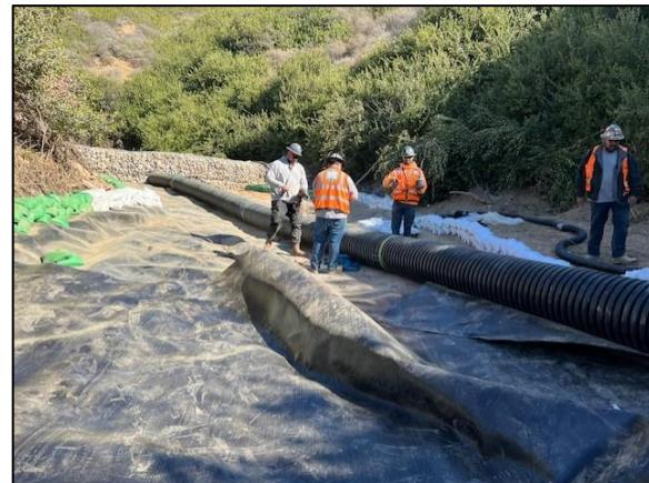
*Completion of New Gabion and Connecting Drainage Pipe in the Upper Section of Klondike Canyon*
