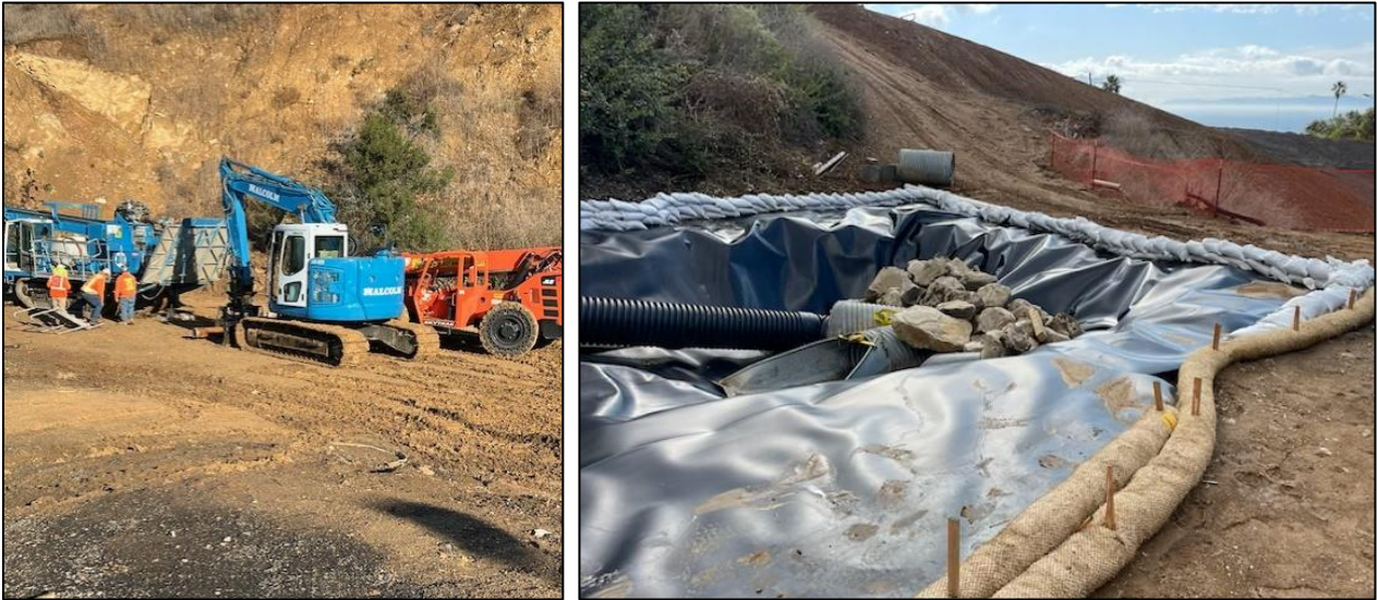
Equipment Setting Up for the Re-Drilling of DDW-8 (Left) and Completed Winterized Interface Between Upper and Lower Klondike Canyon (Right)
