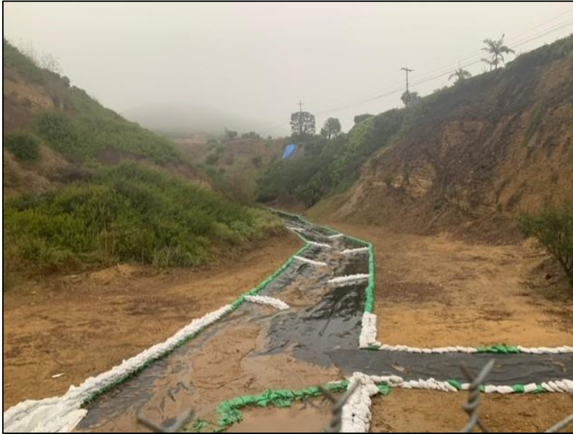
Operation of Winterized Klondike Canyon During Last Week's Storms (Left) and Installation of Additional Liner Securing Measures at Altamira Canyon (Right)
