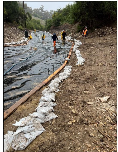
Operation of Winterized Klondike Canyon During Last Week's Storms (Left) and Installation of Additional Liner Securing Measures at Altamira Canyon (Right)
