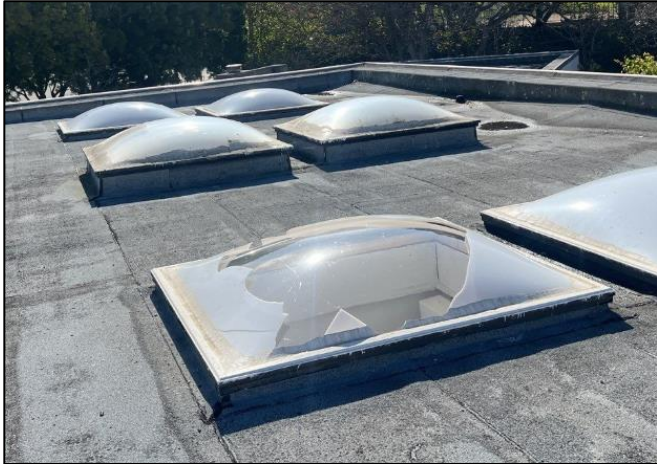
Skylight damage sustained by winds in January, 2025 (left) and view of low points in the existing roof that are causing ponding after rain events (right)
