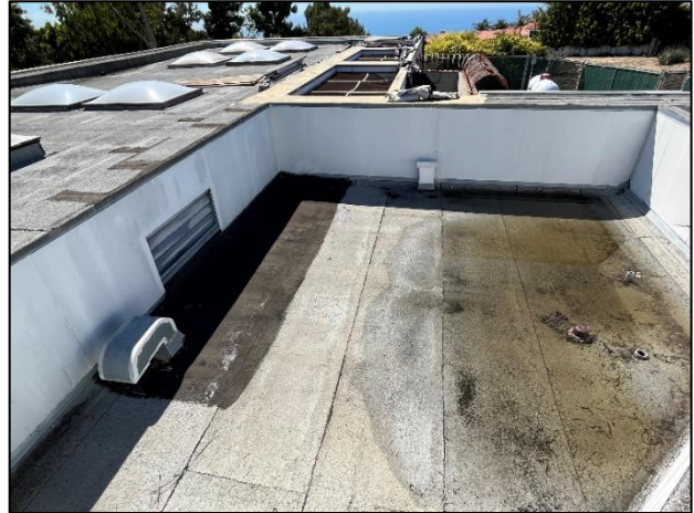
Skylight damage sustained by winds in January, 2025 (left) and view of low points in the existing roof that are causing ponding after rain events (right)
