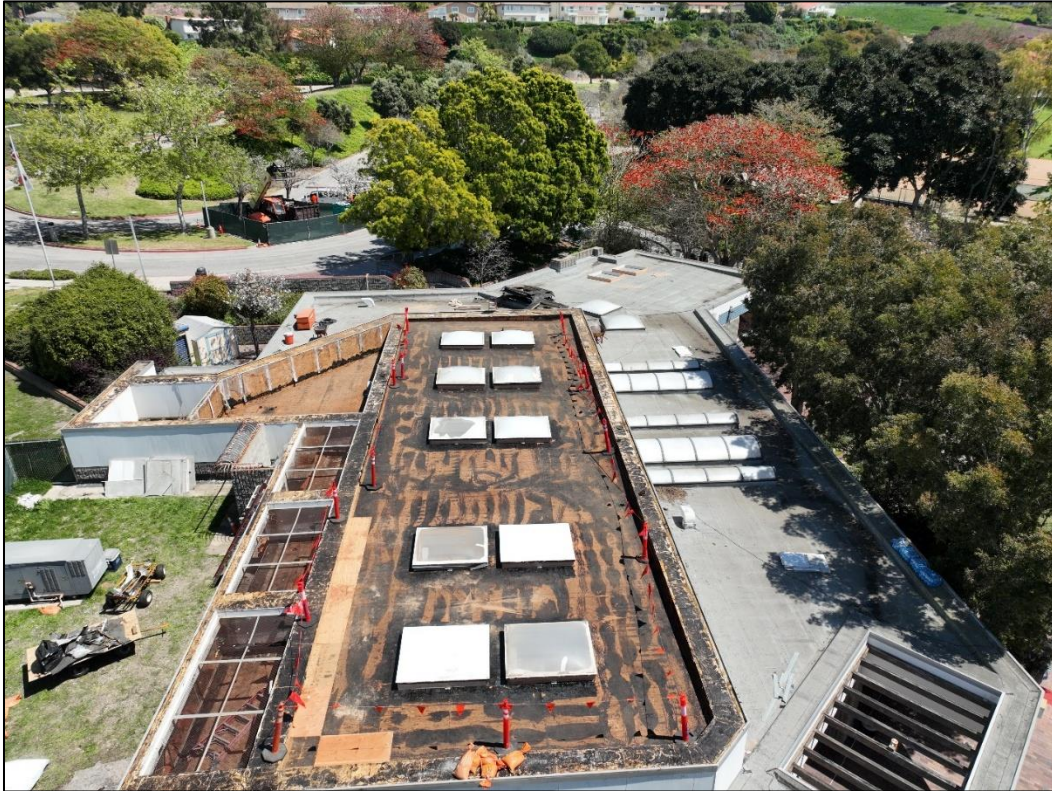
Roof demolition for the Hesse Park Roof Replacement Project.
