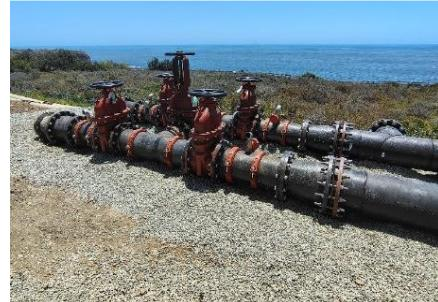
Ongoing land movement in the Portuguese Bend Landslide Complex has damaged these pipelines and caused leaks requiring emergency repairs. In response, LACSD has launched a project to replace the existing rigid steel pipes with more flexible High-Density Polyethylene (HDPE) pipes. Construction began several months ago and is now expected to be completed by the end of the summer.
