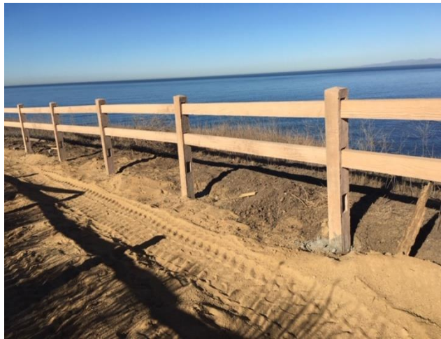
Figure 1 Third row of railing to be installed
