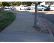
04.25 - Pedestrian Signal Device - Clear Floor Space - Location of pedestrian signal device does not accommodate a level 30" x 48" min.. clear space, centered and parallel to the pedestrian signal push button. (Accessible pedestrian signals shall be located so that the vibrotactile feature can be contacted from the level landing serving a curb ramp, if provided, or from a clear floor or ground space that is in line with the crosswalk line adjacent to the vehicle stop line.)
