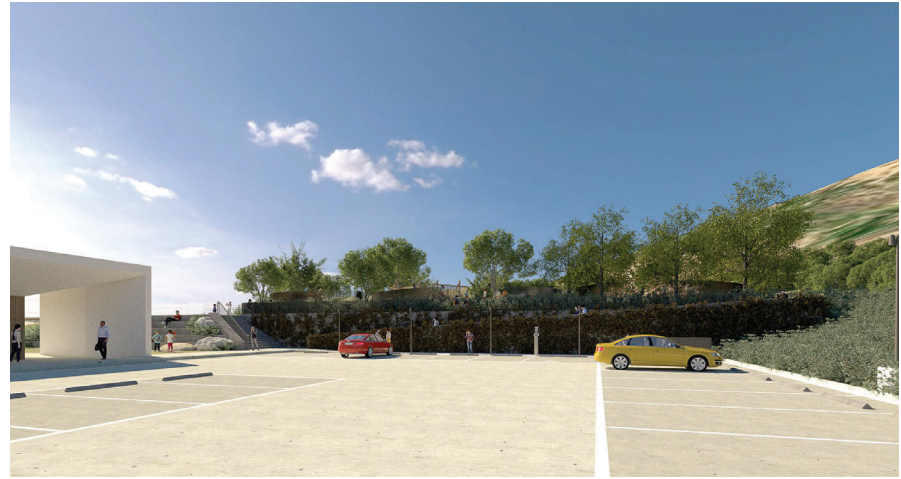
LOOKING EAST FROM PARKING TO ADA RAMP
