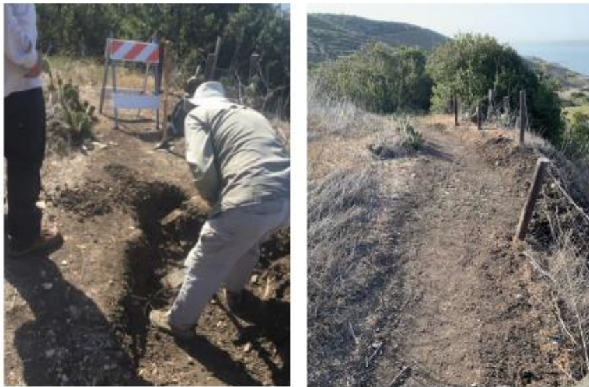
Volunteers are seen above on the left using fill dirt and compacting the trail. Picture on the right depicts the condition of the trail after work was completed.
