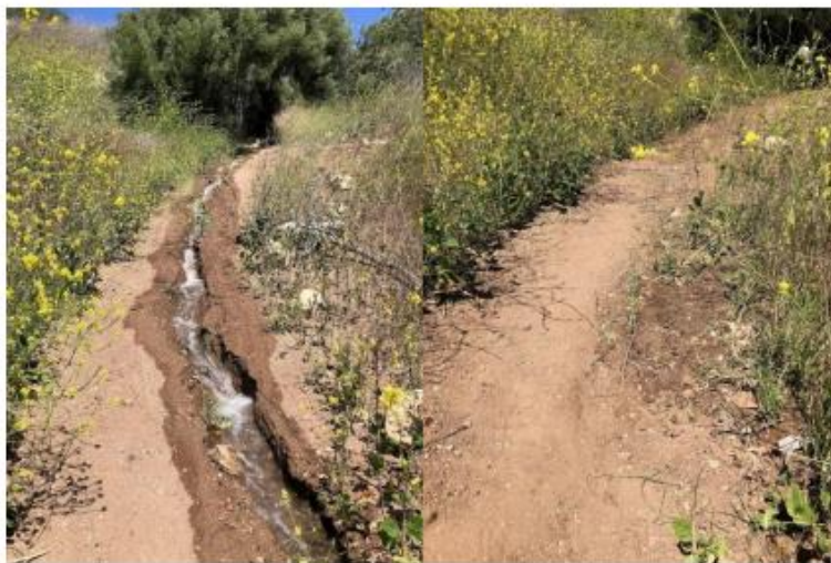
Water flowing onto Vanderlip Trail resulting in rutting on the trailbed prior to it depositing on the adjacent habitat. The picture on the right was taken after trail work was completed to reshape the grade dip and fill in ruts.
