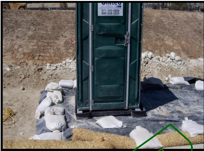
Spill containment for portable toilets
