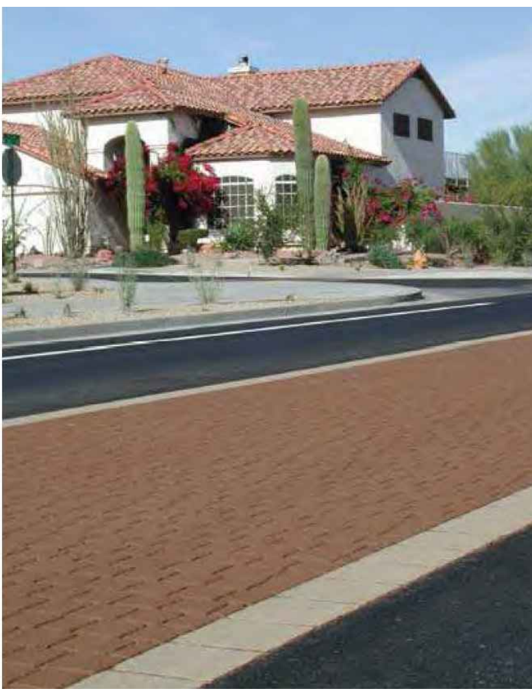
CROSSWALK TREATMENT ( COLOR CONCRETE AND HOT ASPHALT STAMP)
