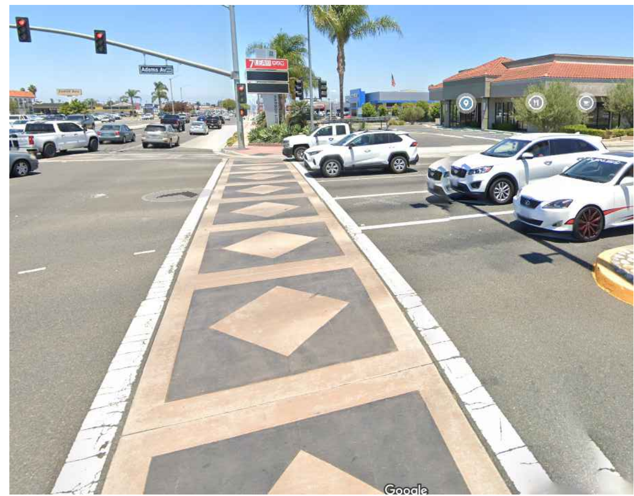
CROSSWALK TREATMENT ( COLOR CONCRETE AND HOT ASPHALT STAMP)
