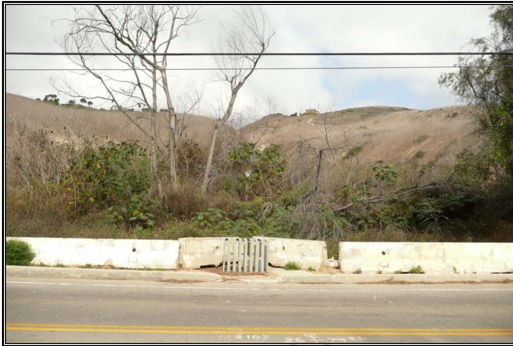
Photo 2: View north up San Ramon Canyon from W. 25 th Street. Existing storm drain inlet structure in foreground.
