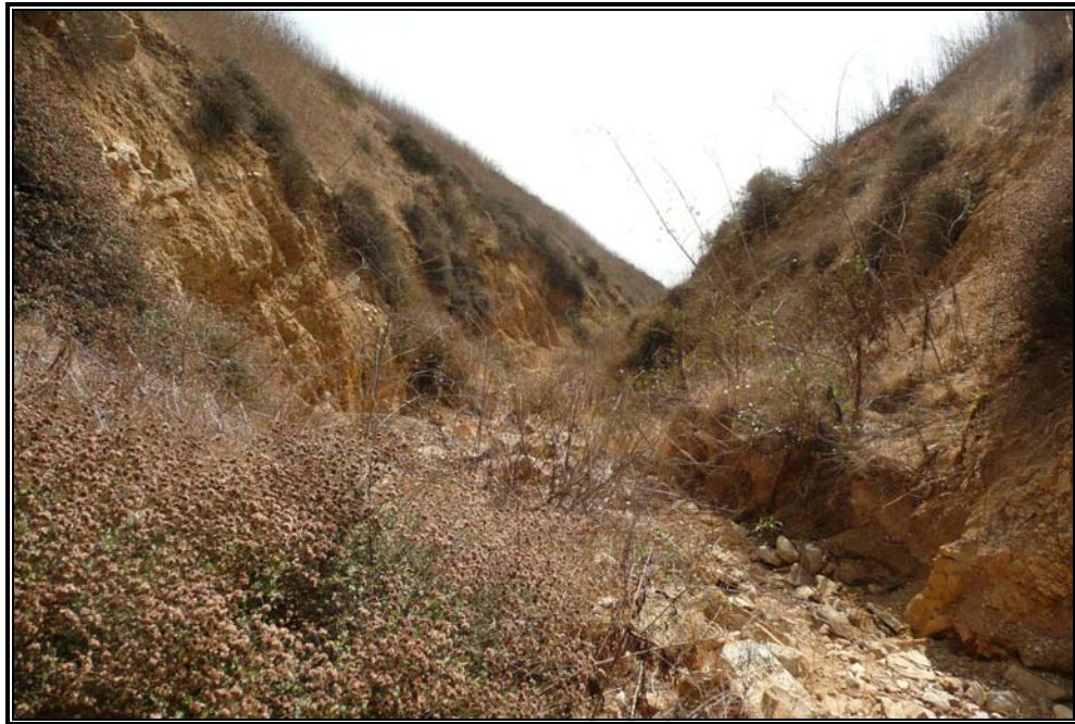
Photo 7: View south down San Ramon Canyon near buttress fill area.
