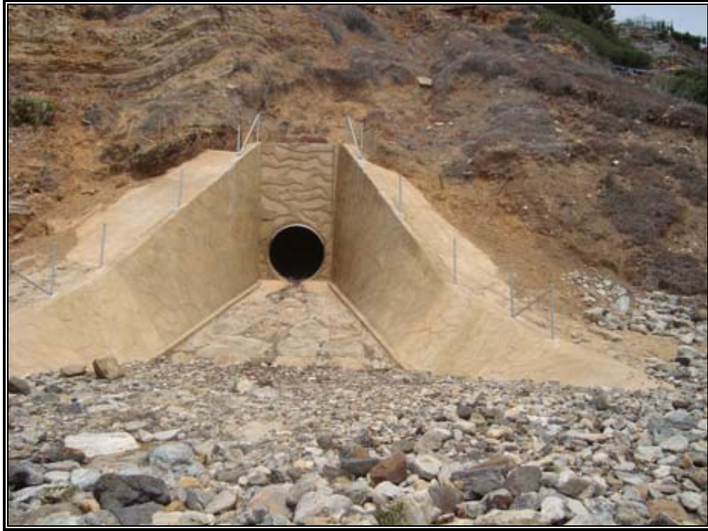
Photo 14: Existing outlet structure for McCarrell Canyon storm drain.
