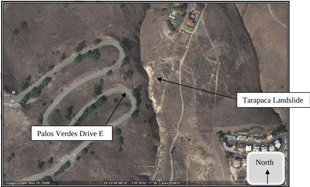
Photo 4: Aerial view of San Ramon Canyon
