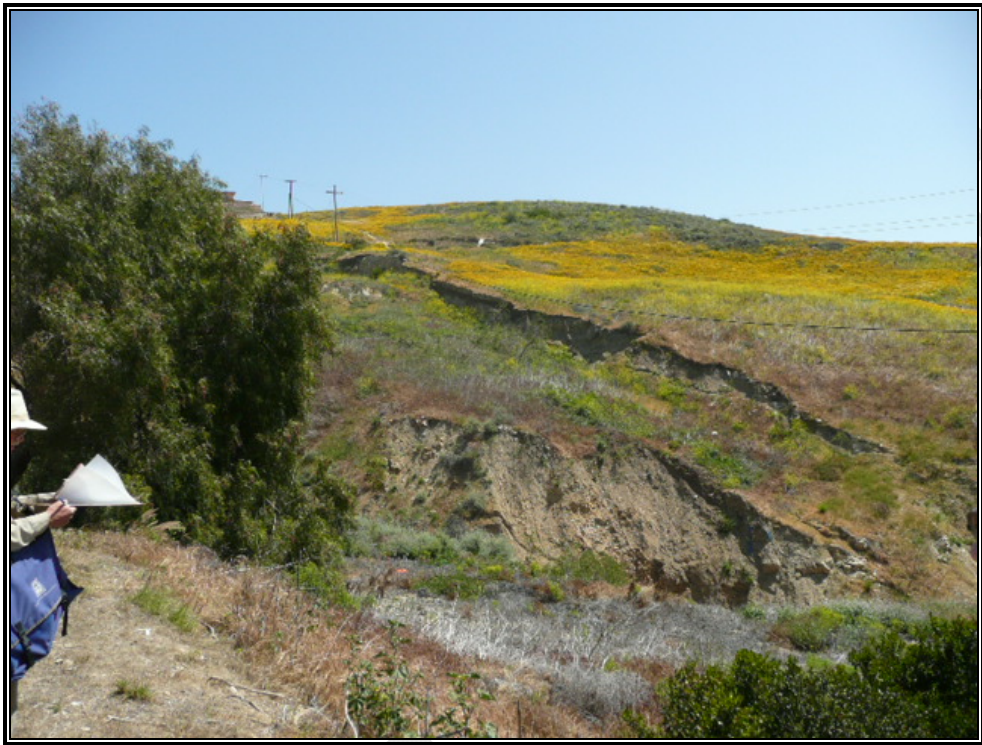
Photo 3: View from PVDE toward the east side of Canyon toward Tarapaca landslide.
