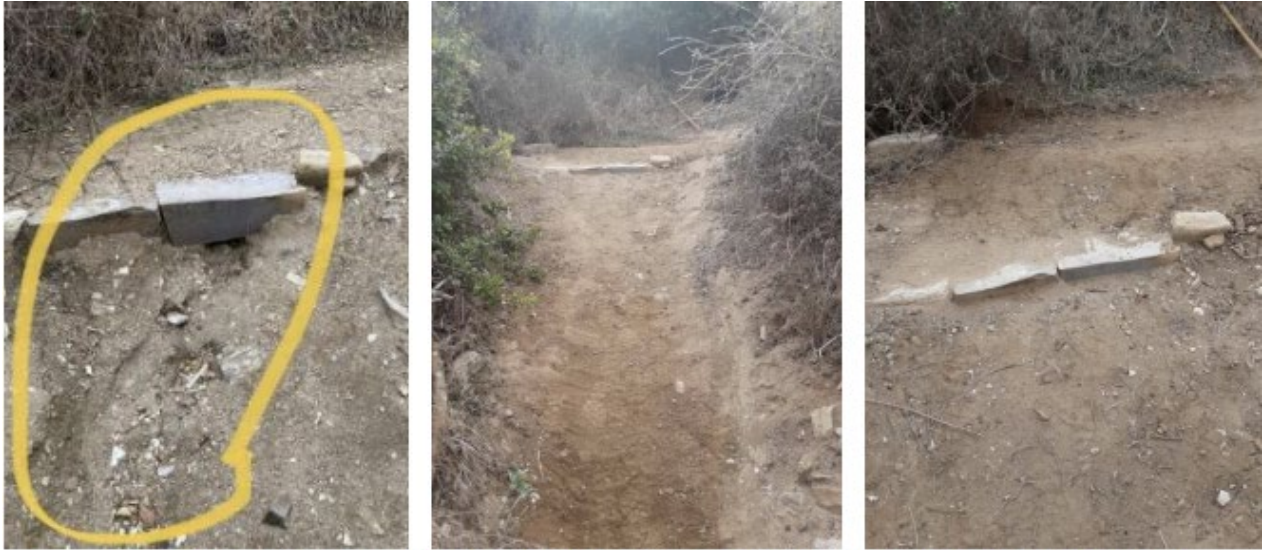
Before (left) and after (center and right) picture of the uppermost rock steps on Sea Dahlia Trail.
