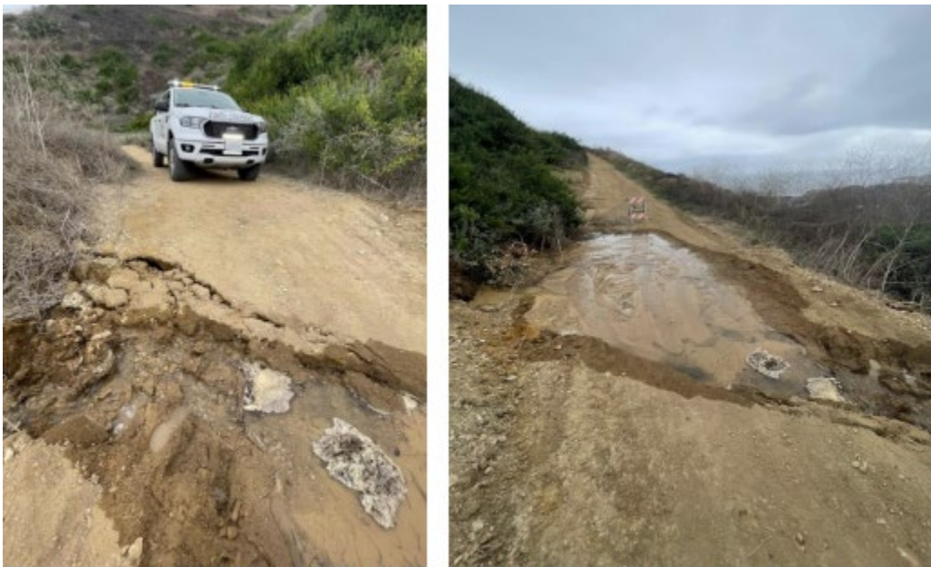
The water main break (left) and the damage on Burma Road Trail is depicted (right).
