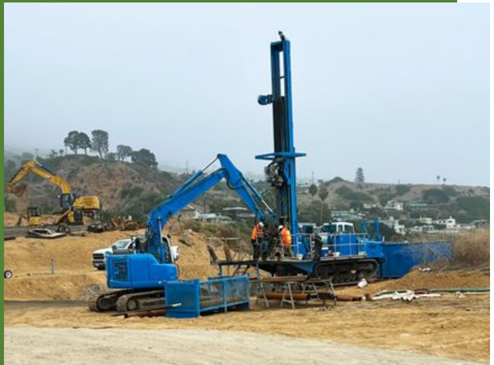
Portuguese Bend Landslide Mitigation Program Deep dewatering wells (Photo of drilling process)
