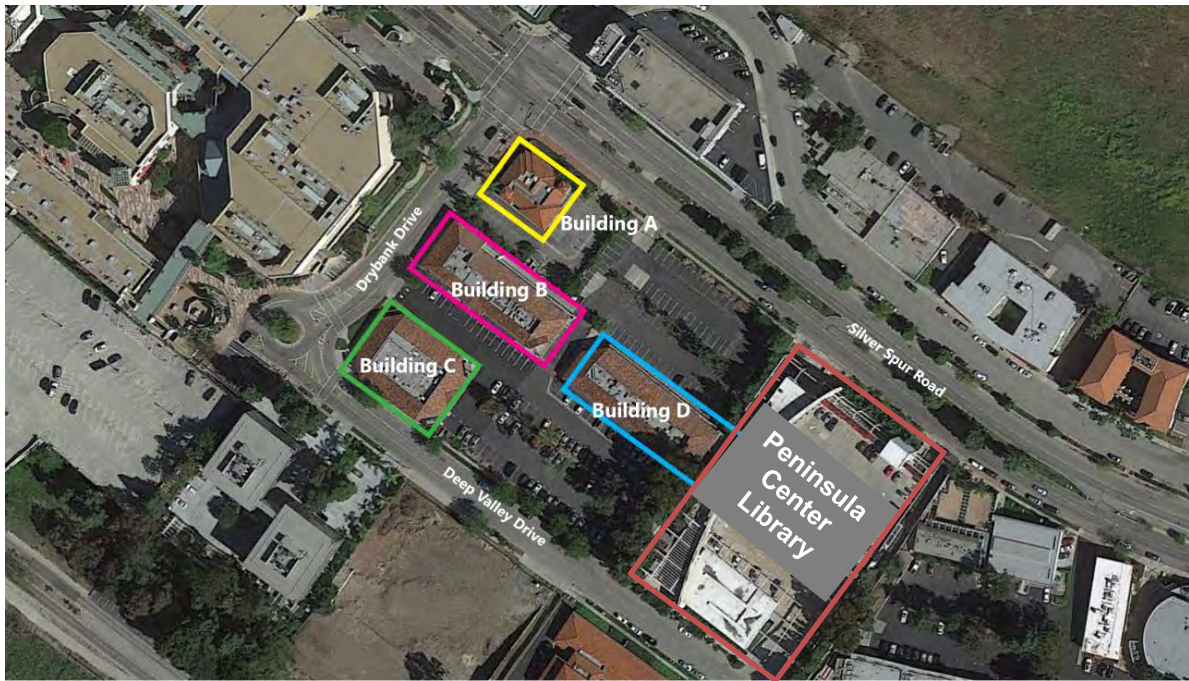
Figure 1 – Existing Project Site
